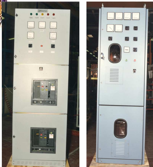
Switching Electrical Panels Network / Group and Command for Generator E.P.
