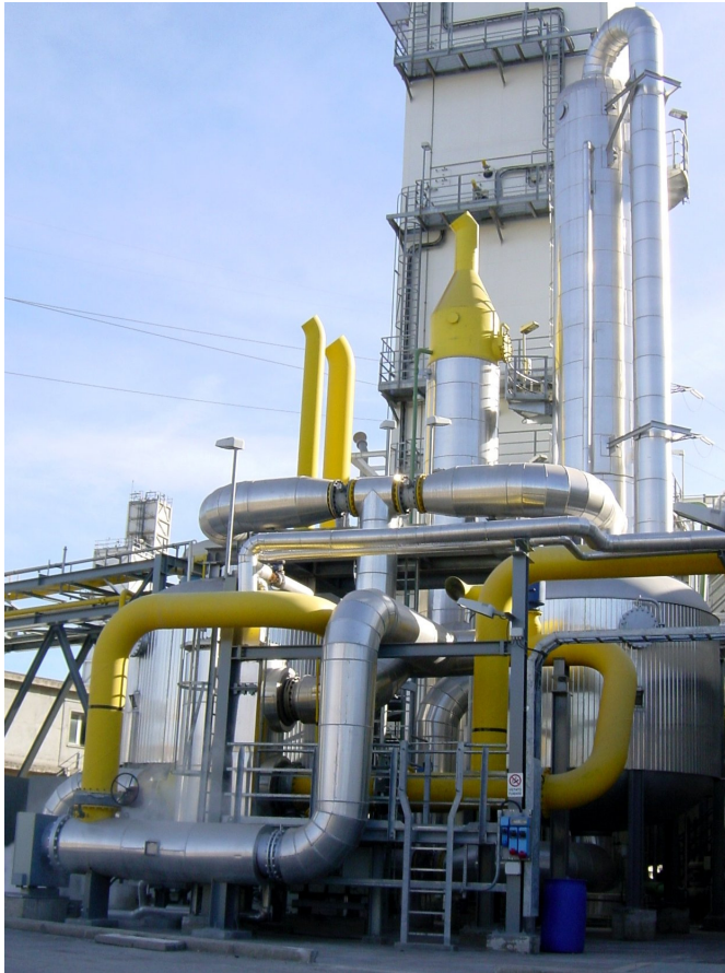
Plant oxygen production
