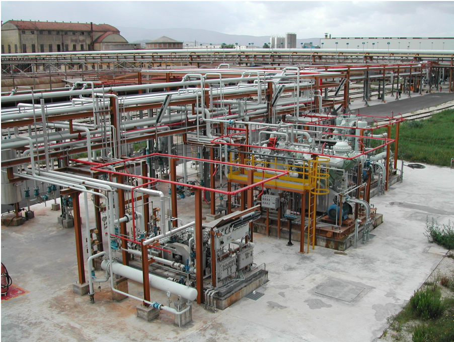
Plant handling and storage liquid propylene
