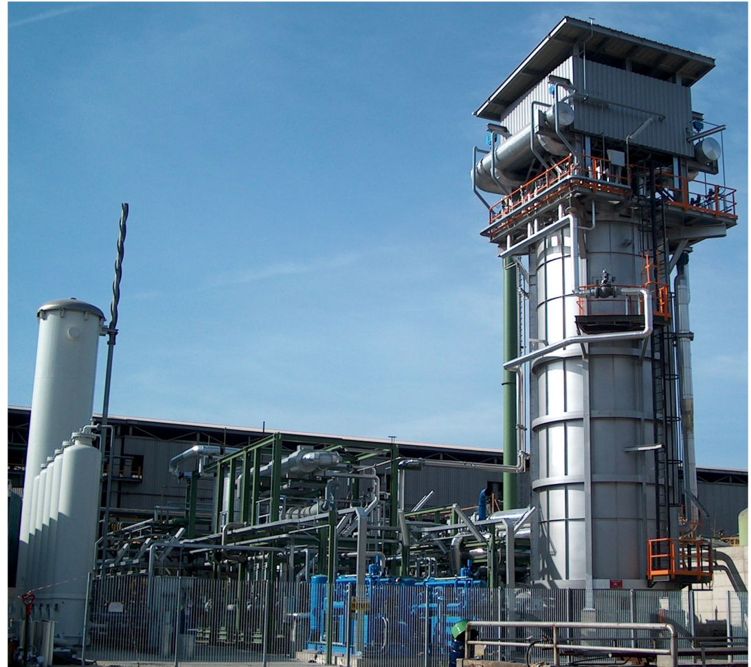
Skid Reducing and Metering Station
